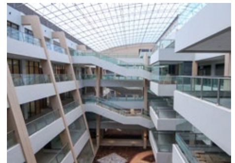
This is a six-storey building including a basement, and covers a plinth area of 13,500 square meters.
